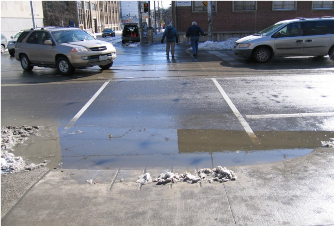
Figure 3: Curb cuts encourage winter accumulations of snow, ice and water. The photo depicts the accumulation of slush and water in the curb cut at the bottom of the photo.
